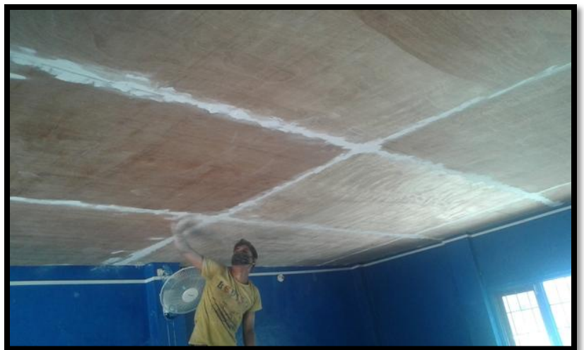
Joints are filling with Putting
